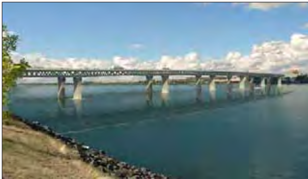
Exhibit 11 Composite Deck Truss
