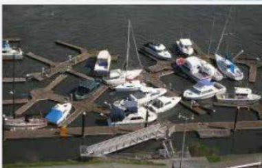
Marina damage near Chetco River, Ore., following wave surges from the March 11, 2011 tsunami off the coast of Japan. Photo: U.S. Coast Guard
